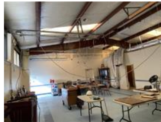
1 st week of renovations
